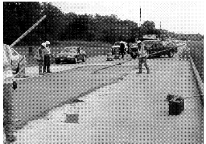
(a) During Paving.
