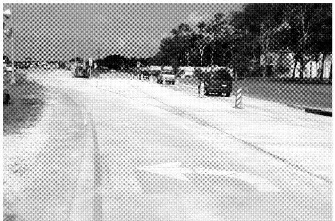
(b) During Curing.
