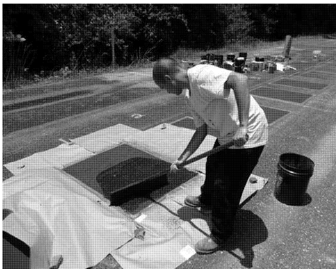
Fig. 2. Placing an Asphalt Sealer with a Squeegee.
