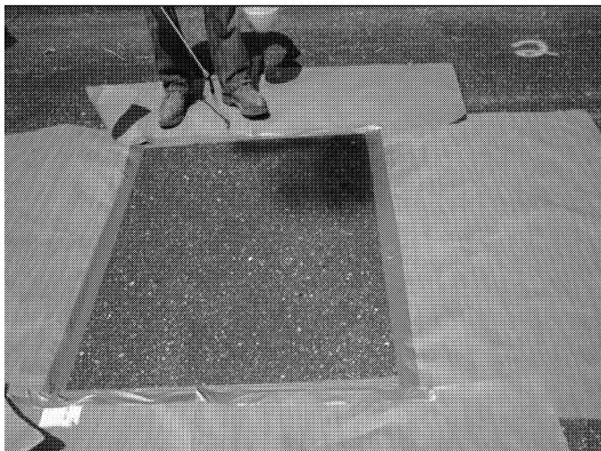
Fig. 1. Applying a Surface Treatment with a Garden Sprayer.
