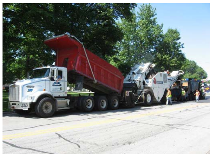
Fig. 3. Construction Train (left to right: Dump Truck Delivering Hot-Mix Asphalt, Material Transfer Device, and Spray Paver).
