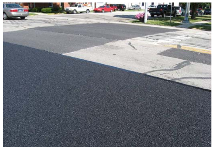
Fig. 4. Finished Wearing Course.
