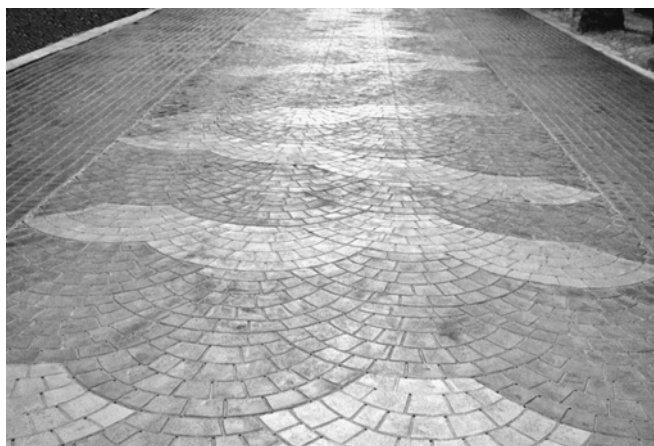
Fig. 2. The Finished Surface of JWS Structural Pervious Air-Circulated Aqueduct Concrete Pavement.
