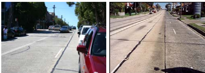
Fig. 3. Local Concrete Roads in Chatswood (left) Built in the 1930s Take Large Numbers of Light Vehicles, Moderate Number of Buses, and Limited Numbers of Heavy 6-axle Vehicles. The Princess Highway (Right) of Similar Age Takes Significantly Higher Heavy Traffic.
