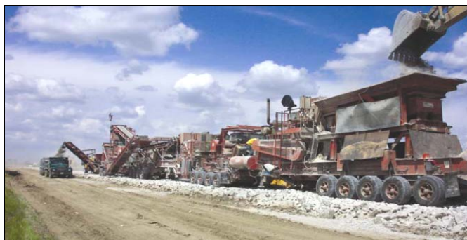
Fig. 8. A View of a Paving Train in Europe for Insitu Recycle Existing Pavements [24].
