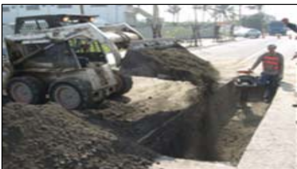
Fig. 2. Test Pit Excavation.
