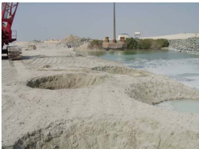
Fig. 9. Dynamic Compaction Craters.
