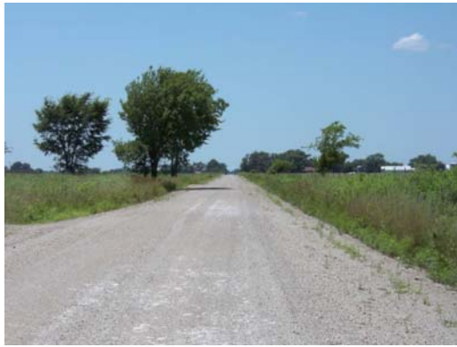
Fig. 1. Photographic View of the Test Road Before Construction.
