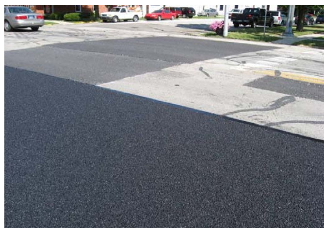
Fig. 4. Finished Wearing Course.
