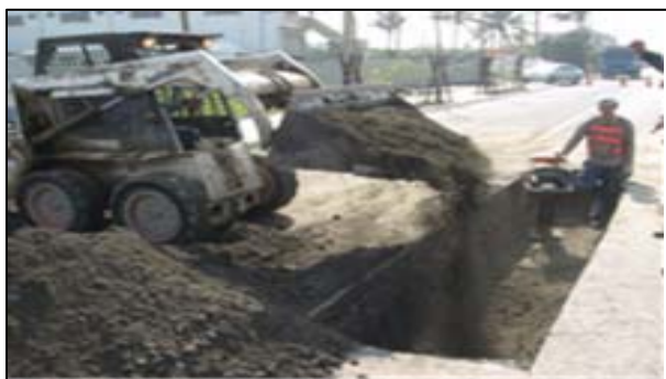
Fig. 2. Test Pit Excavation.
