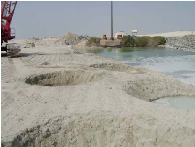
Fig. 9. Dynamic Compaction Craters.
