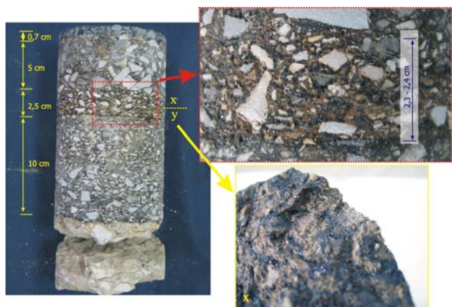
Fig. 7. Core 3a – a 2.5 cm Thick, Pumice-structure-layer at the Depth of Approx. 6 cm. The Cross-section of the Layer shows the Results of Aggregate Degradation and Insufficient Amount of Asphalt Binder.
