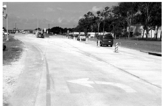
(b) During Curing.
