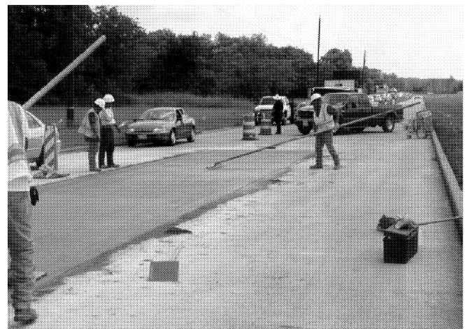
(a) During Paving.
