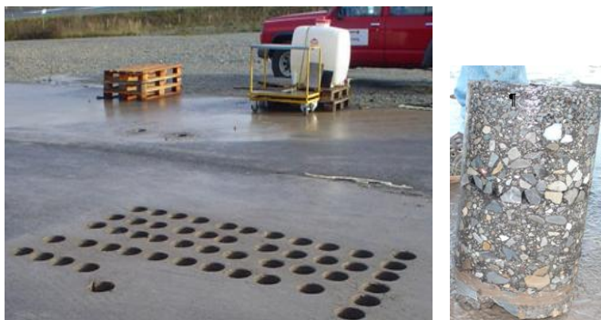
Fig. 5. Coring of Pavement 3.
