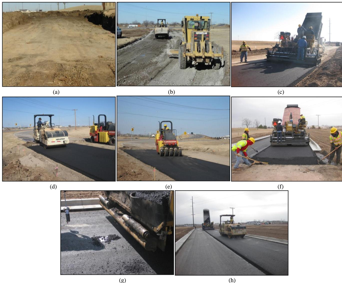
**Fig. 1.** (a) Right of Way (Natural Subgrade), (b) Mixing CKD With Subgrade, (c) Laydown of S3-25 Layer (South Lane), (d) Compaction of S3-25 Layer With Steel Drum Roller, (e) Compaction of S3-25 Layer With Rubber-tire Roller, (f) Laydown of S4-0 Layer (South Lane), (g) Placement of Paper During Laydown of S4 Layers, and (h) Laydown and Compaction of S4-0 Layer (South Lane).
