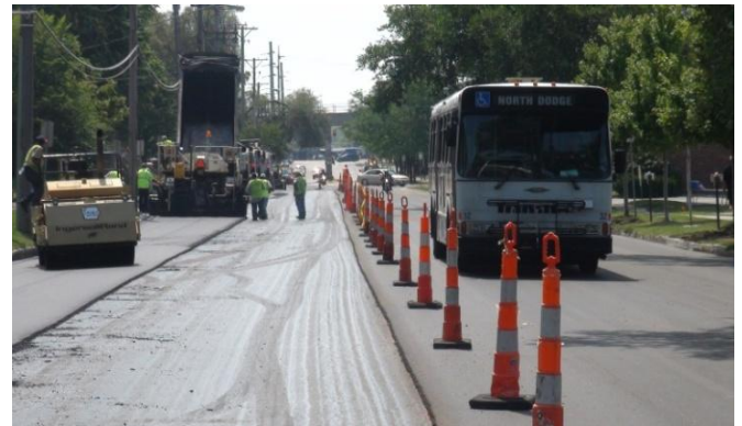
Fig. 8. WMA Pavement with the New PE Wax-based Additive on Capitol Street in Iowa City.
