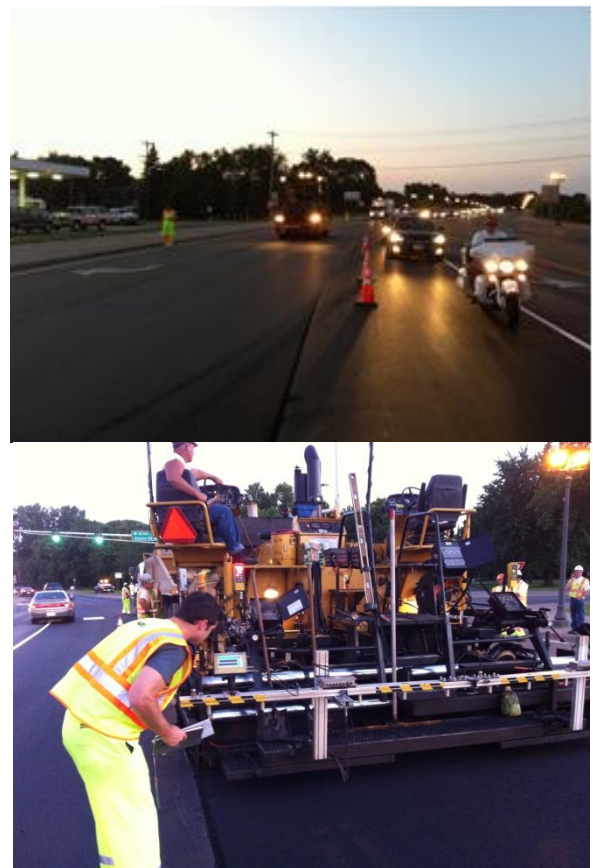
Fig. 11. WMA Rehabilitation Project on TH 169 State Highway in Champlin, Minnesota.
