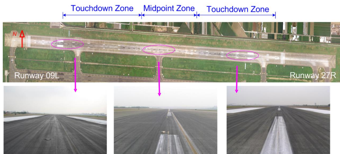
Fig. 1. Rubber Deposits at the Kaohsiung International Airport (KIA).
