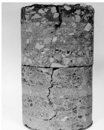
Fig. 4. Top-down Reflective Cracking [34].
