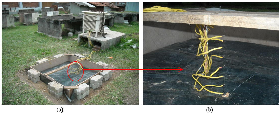
Fig. 7. Thermocouple Arrangement in the Slab (a) Formwork Placed on Thick Polythene Sheet, (b) Thermocouples Attached to the Formwork Using non-elastic and Thermoplastic Wire.
