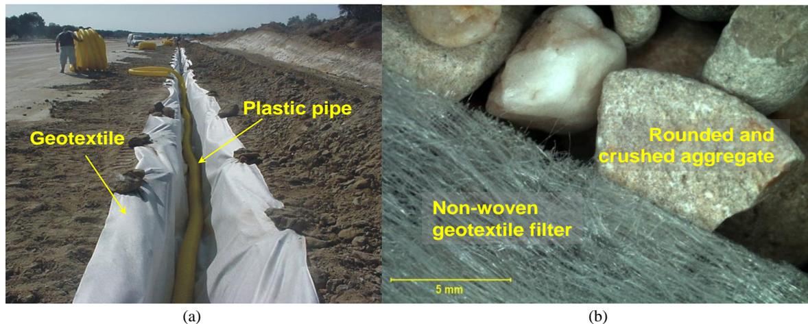
**Fig. 1.** Conventional Drainage: (a) Trench Drain Under-construction and (b) Main Construction Materials Used.
