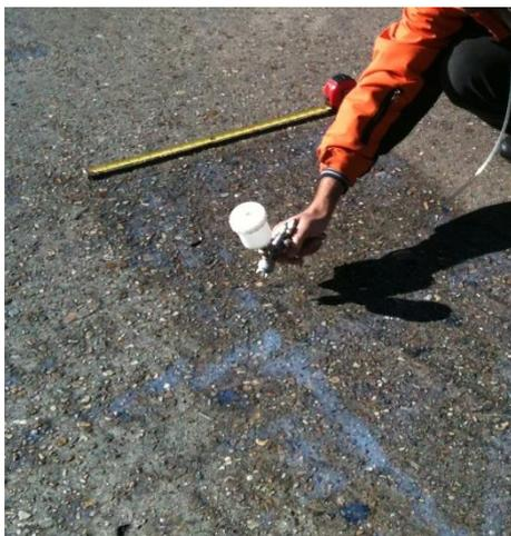
**Fig. 2.** TiO<sub>2</sub> Spray Coat Application.
