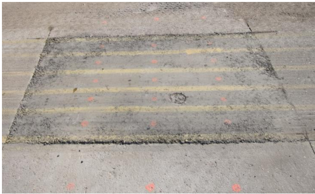
Fig. 7. Example of Repair after Trafficking
