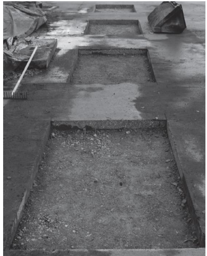
Fig. 5. Excavated Field Repairs Prior to Asphalt Placement.
