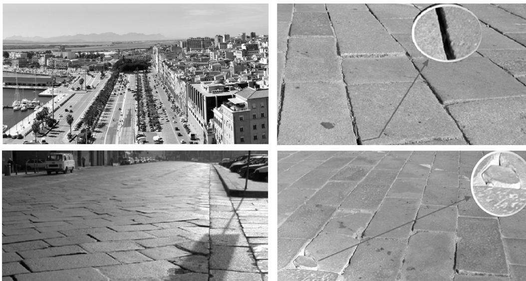
Fig. 2. The flagstone pavement on the Cagliari waterfront and typical distress.
