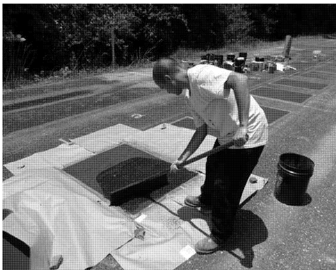
Fig. 2. Placing an Asphalt Sealer with a Squeegee.
