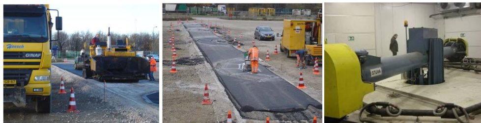
Fig. 10. Left to Right; Test Slab Construction Using Regular Road Building Equipment, Retrieval of Test Slabs, and View on STUVA's APT.
